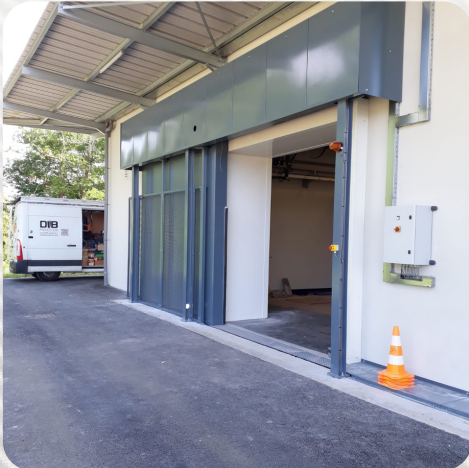
Heavy door with motorized folding threshold
