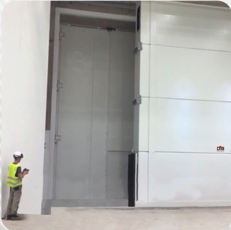
Rolls Royce heavy armoured door 380 tons - 12m*10m*1m
