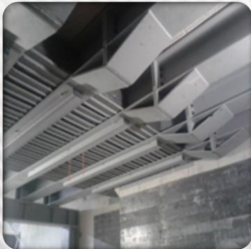
*Long-span lead support beams*
